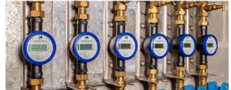
PoC: digital water meter with acoustic noise detection
